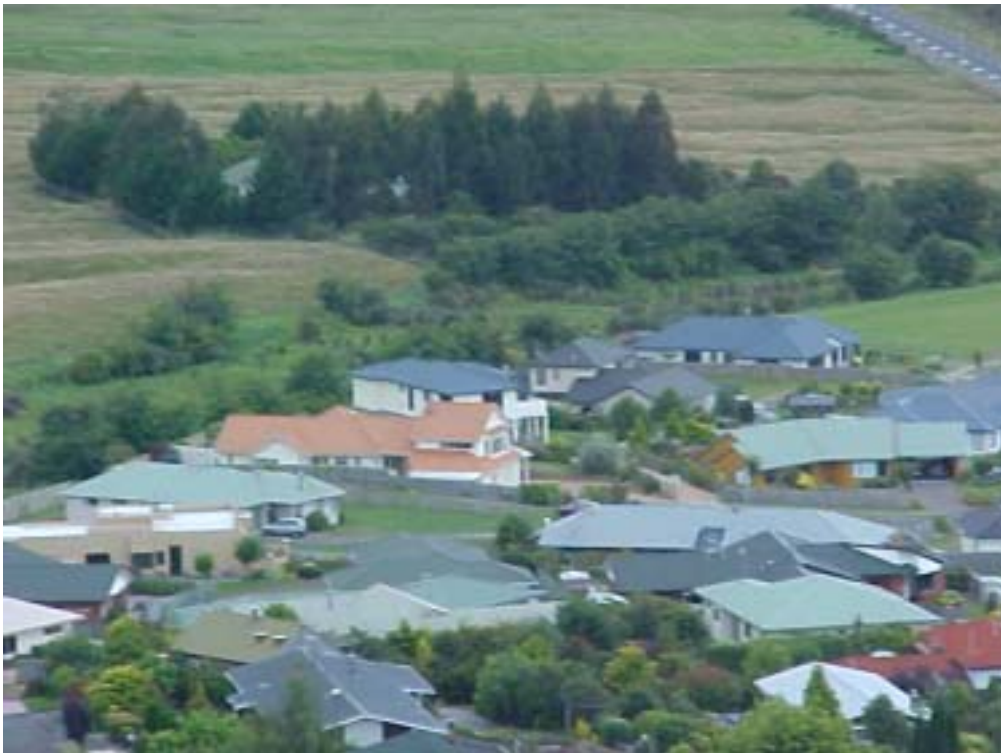
Figure 3 Aerial Views of Acacia Bay, Taupo, SBR Treatment Plant (within the grove of trees)
